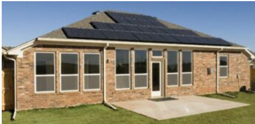
Figure 1: PV array on the roof of Ideal Homes' Zero-Energy Home in Oklahoma City, OK [1]
