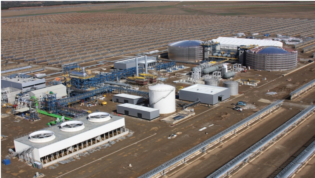
Figure 2: View of the power block in Andasol-1
