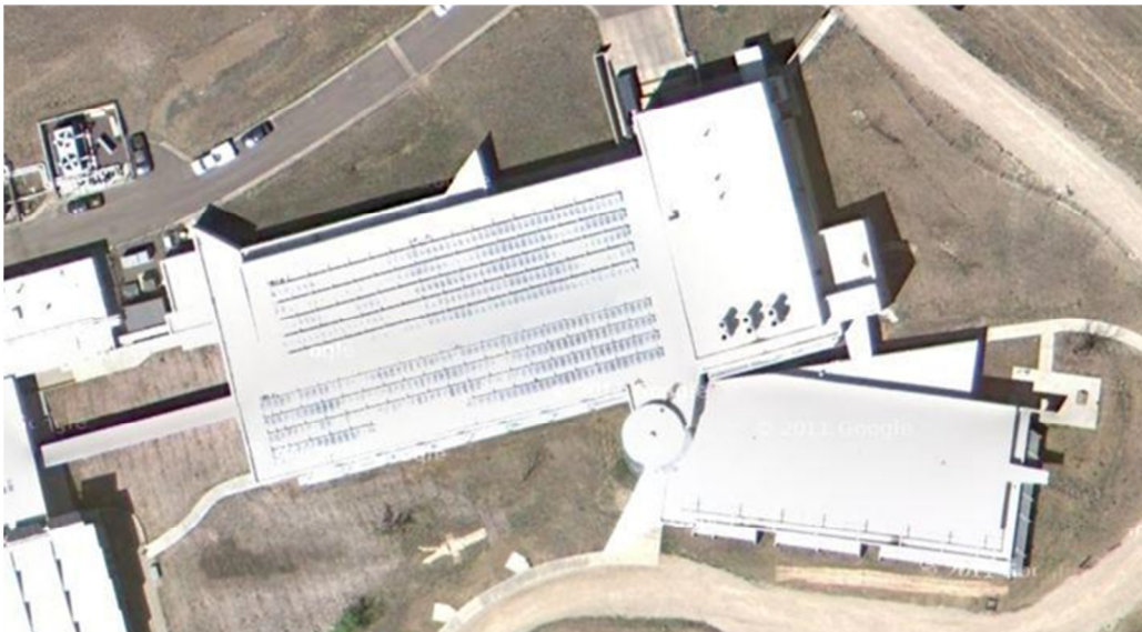
Figure 1: Aerial view of the PV array on the S&TF roof [1]
